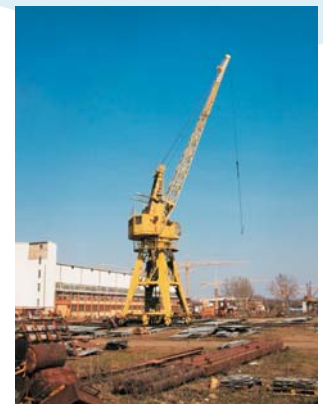
Work Site Monitoring
